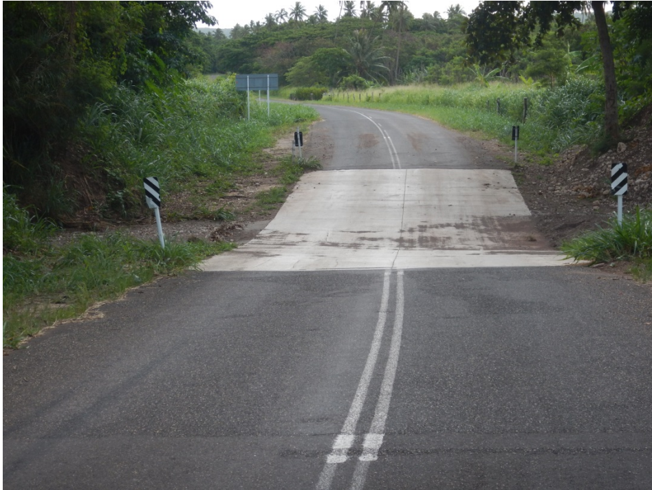
Figure 28 Lakenasua Unvented Drift Crossing
