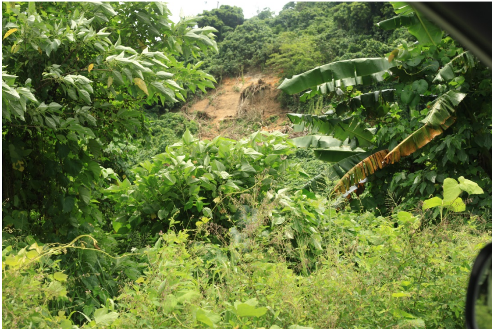
Figure 22 Slope instability above Ring Road
