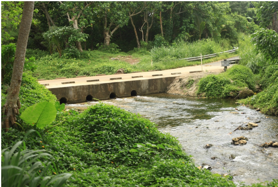
Figure 21 Side view showing vented drift
