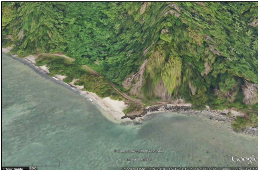
Figure 52 Assen Point Road
