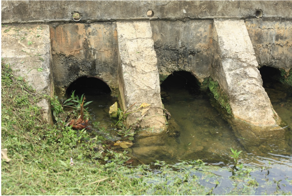
Figure 18 Very Small Culverts
