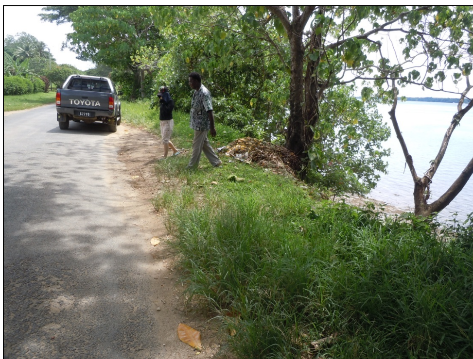
Figure 44 Erosion near Coral Quay
