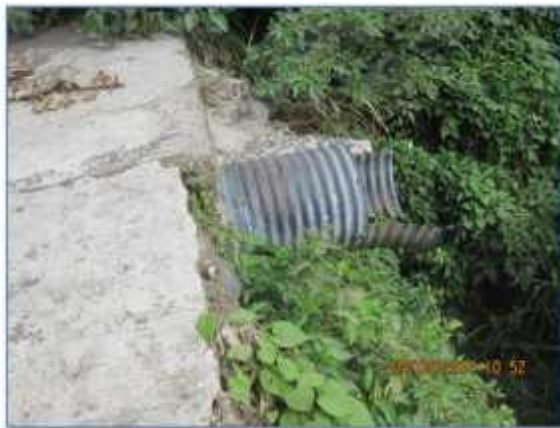
Figure 32. Cross drainage poorly maintained
