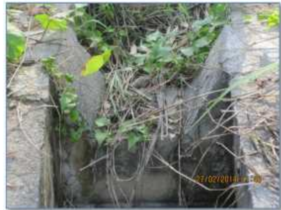
Figure 32. Cross drainage poorly maintained
