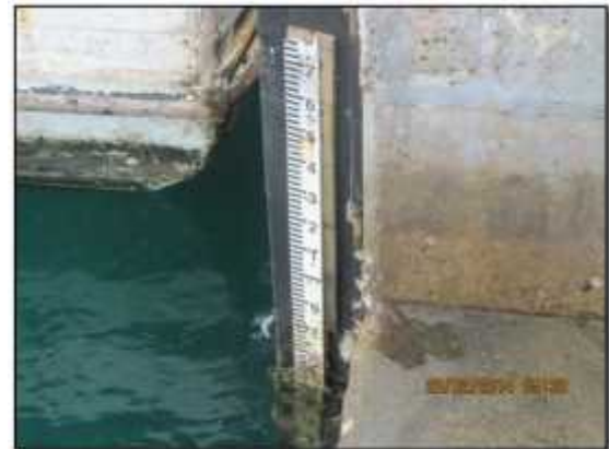
Figure 51. Wharf with low freeboard at high tide. Tide Gauge
