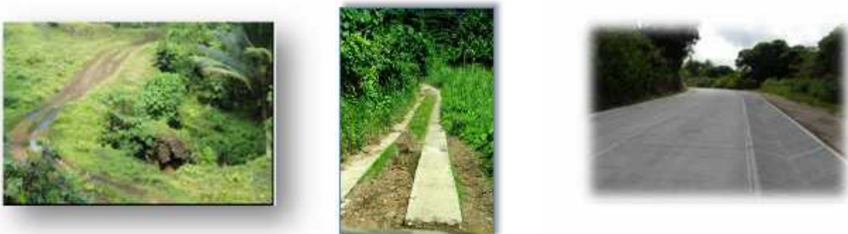
Figure 54. Vulnerable steep muddy road, concrete strips and Climate Resilient road
