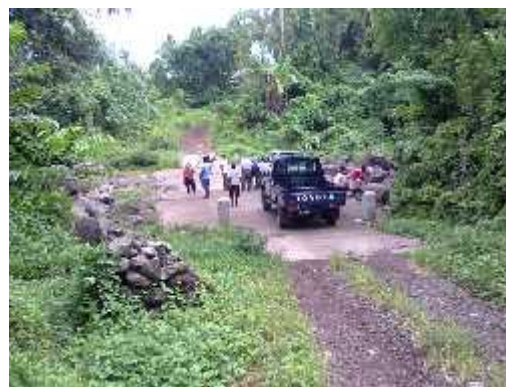
Figure 35. Low Level Crossing with flow and drift with guideposts
