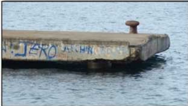
Figure 51. Wharf with low freeboard at high tide. Tide Gauge
