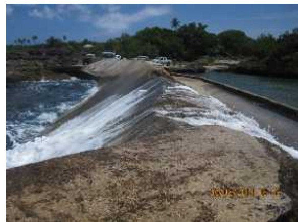
Figure 51. Wharf with low freeboard at high tide. Tide Gauge
