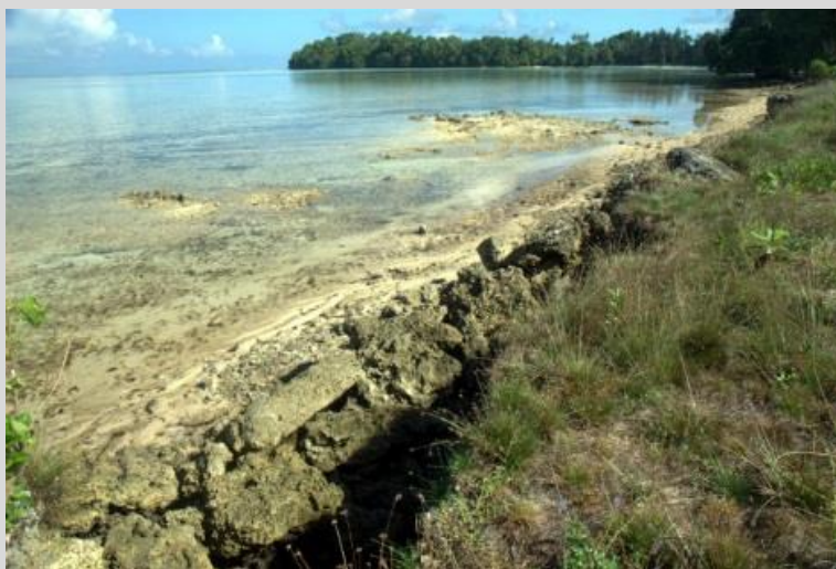
Plate 6: Northern end of Taro airstrip at low tide. Note active erosion behind existing coastal protection rip rap.
