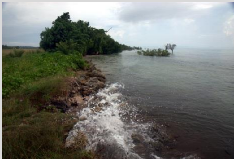
Plate 2: Looking south along the western side of Taro airstrip, in the foreground waves are breaking over existing coastal protection rip rap, and in the background the vegetated buffer along the western side of the airstrip can be seen.
