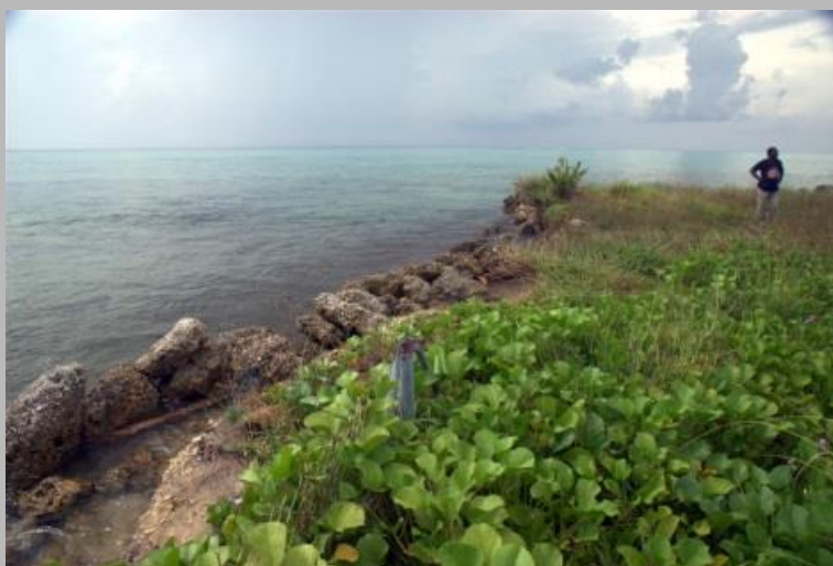
Plate 3: Northern western corner of Taro airstrip at high tide. Note active erosion behind existing coastal protection rip rap.
