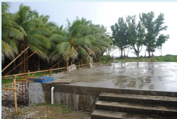
A cistern under construction in Lofeagai, Funafuti
