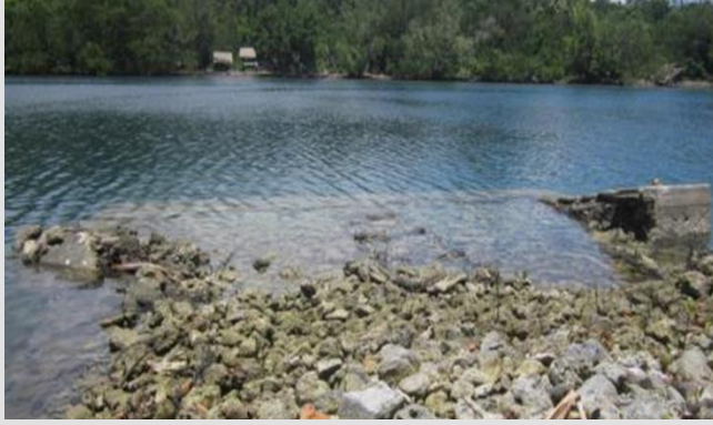
Plate 4: Condition of the existing Lambulambu Wharf in 2012
