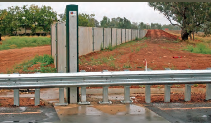
Levee wall, Charleville, Qld Image: Michael Jefferies
