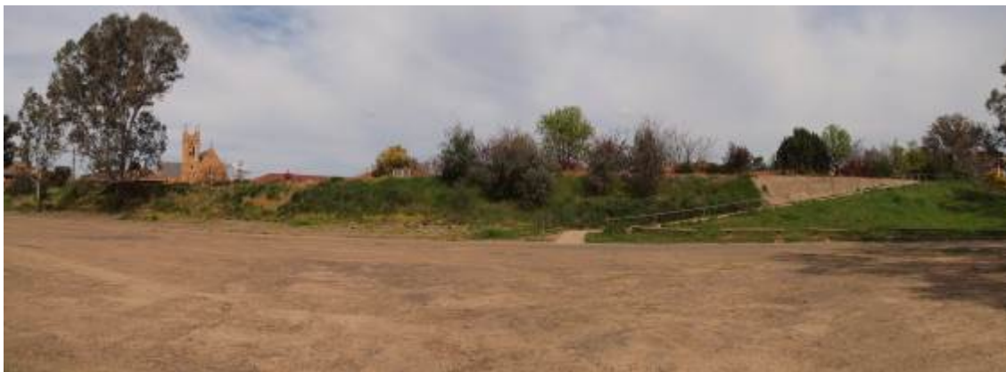
CBD Flood levees, Wagga Wagga
