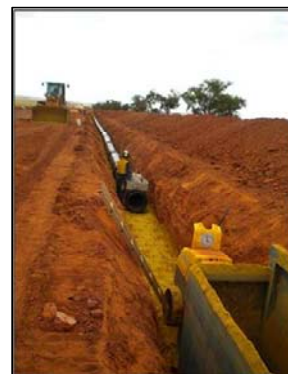
Images: Laying Karara water pipeline (above) and Karara township (top)
