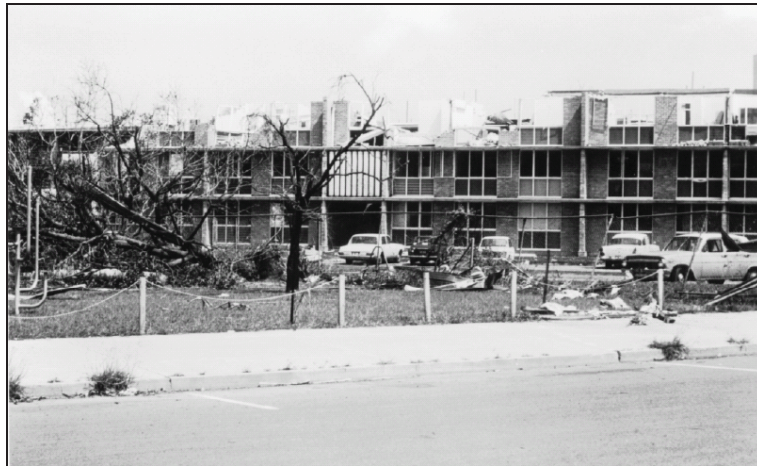
Figure 19: Failure of the top level of a block of flats
