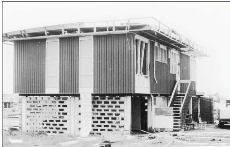
Figure 18: Survival of a house clad in sheet metal
