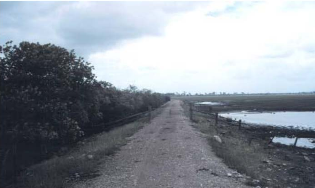
Mangrove growth along pondage bank adjacent to Fitzroy River.
