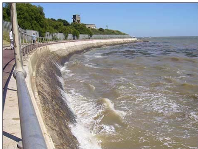
Engineering solutions protect settlements
